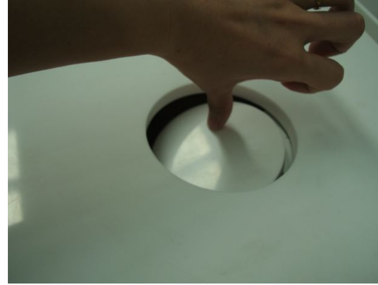
WHITE CORIAN WITH CIRCULAR DISPOSAL UNIT - SPRING LOADED TOP.
